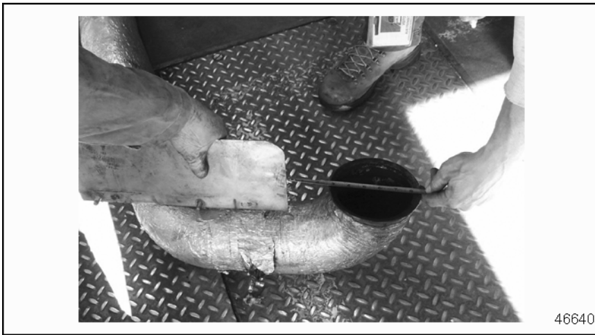
Figure 2 Cutting Inlet Pipe 5.5 in. Below Outlet Centerline
